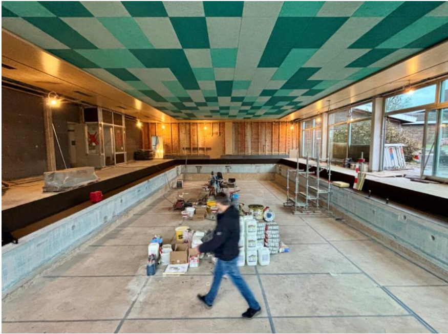
Prepared swimming pool with the pool head cut out and waterproofing ©agrob-buchtal.de
