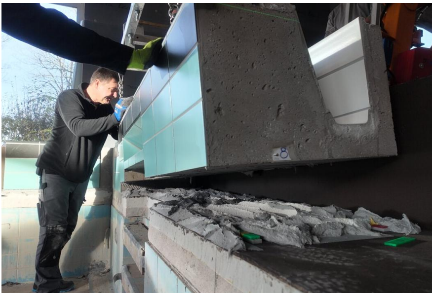
Prefabricated component with integrated rung ladder is hoisted into place. ©agrob-buchtal.de
