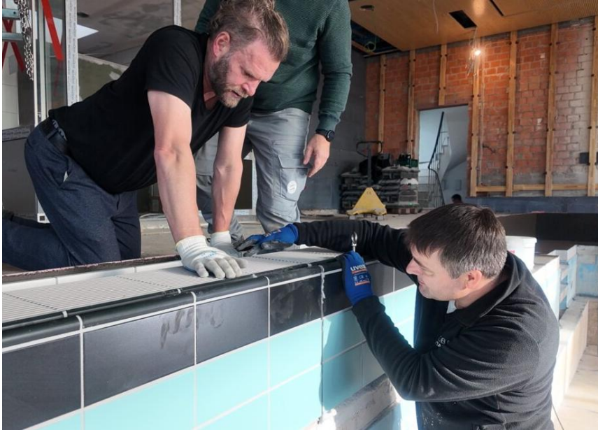
Andreas Kramer (right), Head of Architectural Services at Agrob Buchtal, checks that the CarboCeram prefabricated component fits precisely ©agrob-buchtal.de
